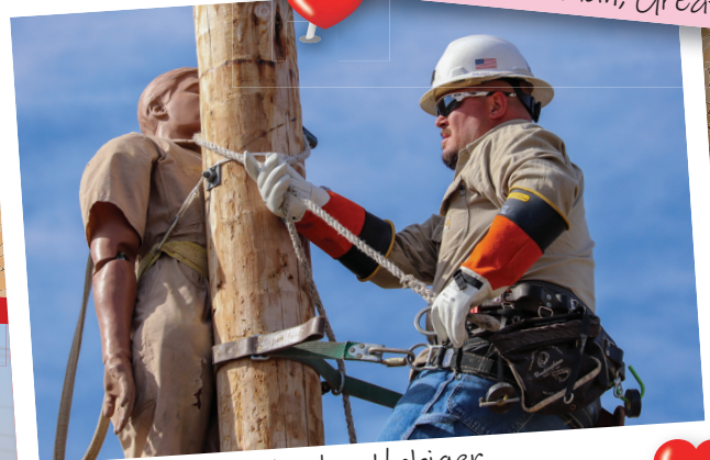
Jordan Habiger Journeyman Lineman, Scott City
